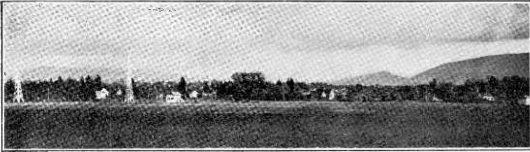
General View. The Aerial and Transmitting Building are on the left and the Hangars on the right.
